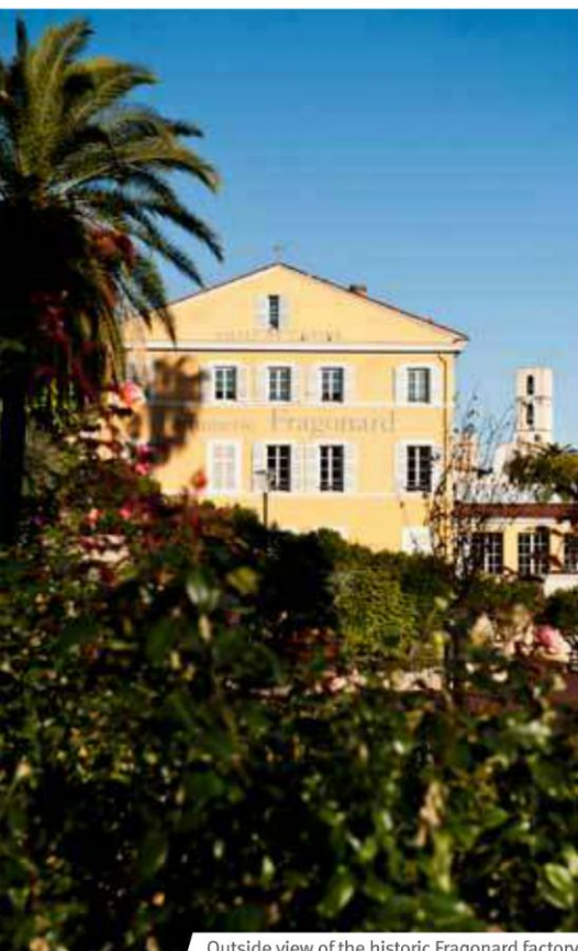
Outside view of the historic Fragonard factory.
